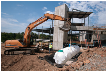
This 1,700-gallon underground cistern stores runoff water from the CSL roof for reuse as flush water.
