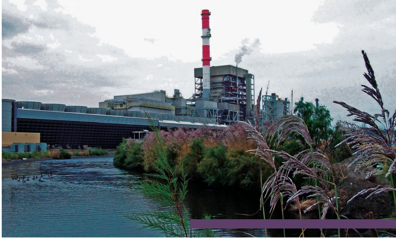
Coal Combustion Residuals (CCR) are a by-product of the creation of electricity.
